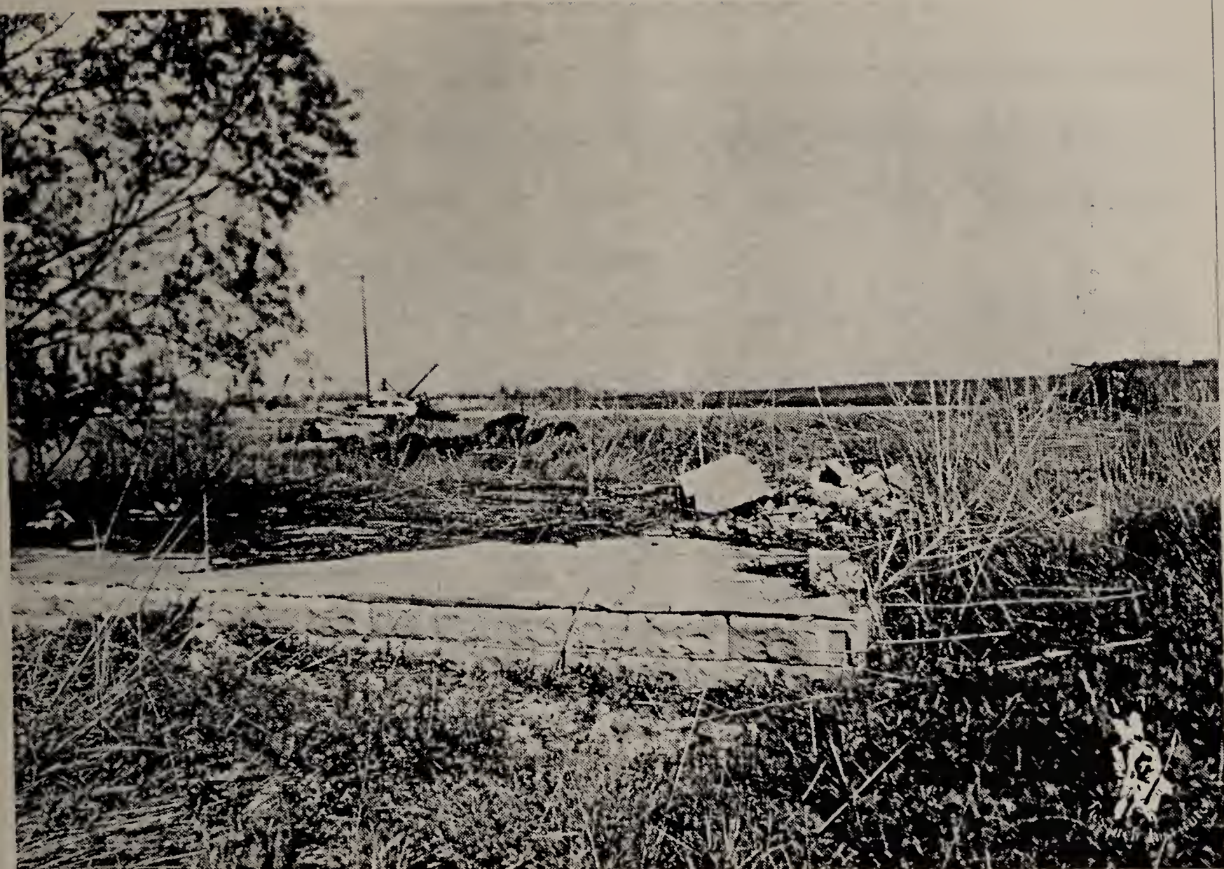
Plate 3. Cement and brick foundation at the George Berry plantation location. This foundation is probably the remains of George Berry Washington's gin. According to local informants, the gin press or gin boiler rested on the foundation. The gin was destroyed by a steam boiler explosion and never rebuilt. The precise date of the explosion could not be determined, but tax records indicate that the gin was extant in 1923.
